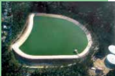
The Forest Lake Reservoir stores recycled water for irrigation and firefighting, and also helps protect habitat in the Carmel River and ocean.
